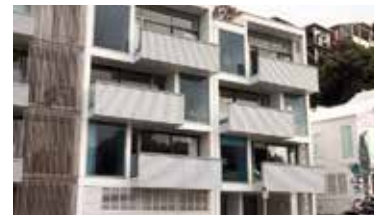
Medium density housing 3-4 storey apartment buildings
