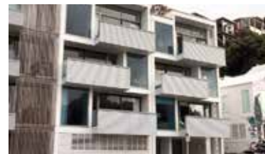
Medium density housing 3-4 storey apartment buildings
